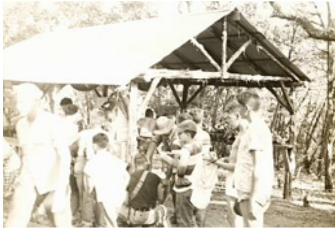
Overnight shelter at Mansfield Dam.
