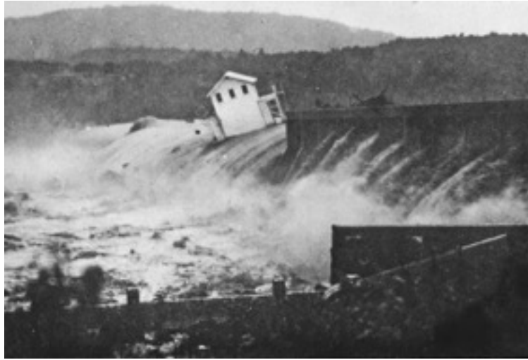
A view of the Austin Dam during the 1935 flood.
