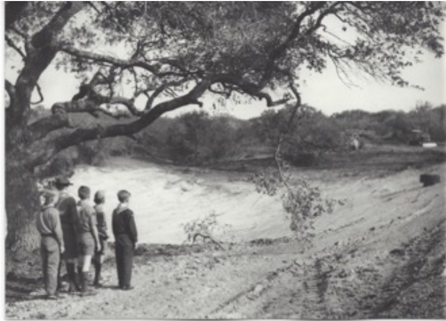
Photo of Lake Allen being constructed on the Green Dickson property in 1967.
